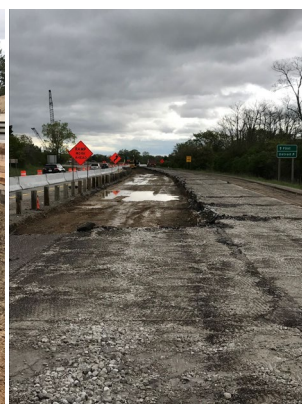
Corporate Dr. Pavement Removal
