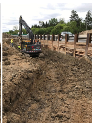
Wattles Rd. Center Pier Retaining Wall
