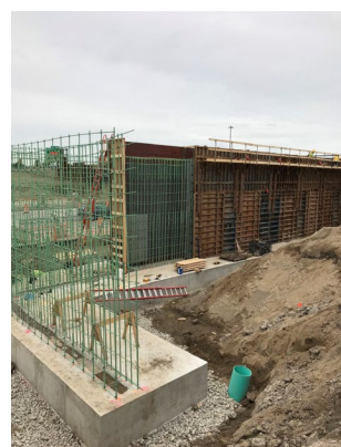
14 Mile Rd. Stem Wall with Forms
