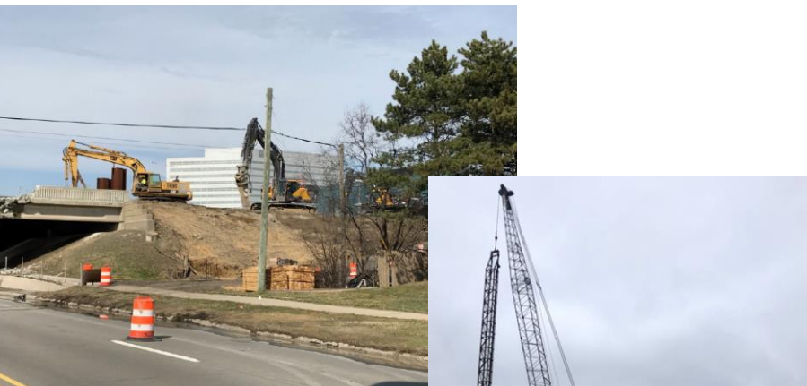
Livernois Bridge Demolition
