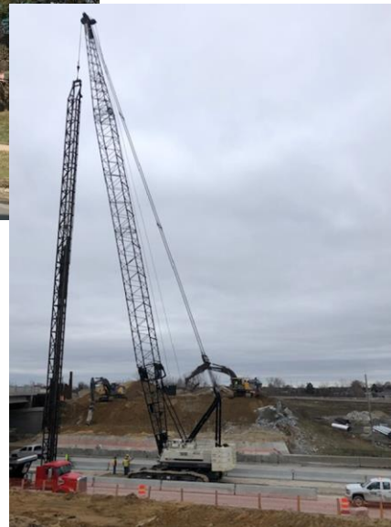
Lifting Pile at Big Beaver
